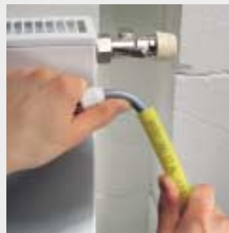
Bending the pipe by hand
